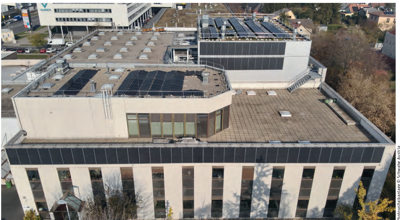
Photovoltaikanlage © Schwabe Austria
